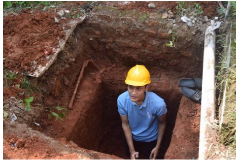
Gambar 4. Galian Sumur Resapan
