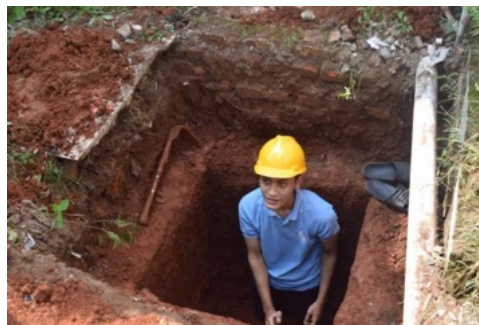
Gambar 4. Galian Sumur Resapan
